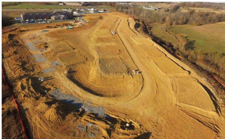
Phillips Brothers moved 40,000 cu. yd. of earth in preparing the 15-acre site for the Robinbrooke subdivision in Elizabethtown, Ky.
